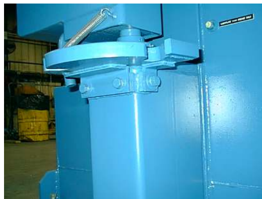
Fig. 2 - 24: Completed Lock Plate Installation
